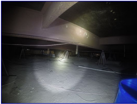
Crawlspace area view.
