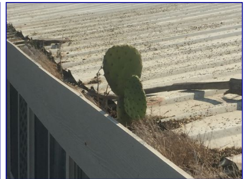
there is a cactus plant growing on the roof of the front enclosed porch.
