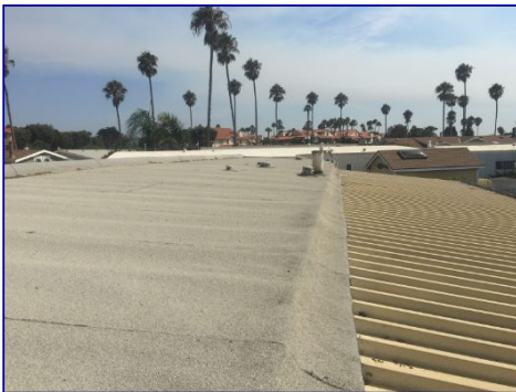
Roof is in functional condition.
